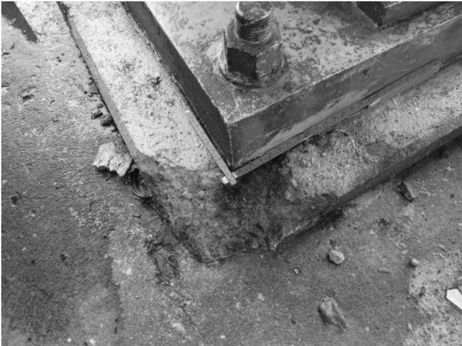
PIER 9 NORTHBOUND BRIDGE UPSTREAM BEARING
