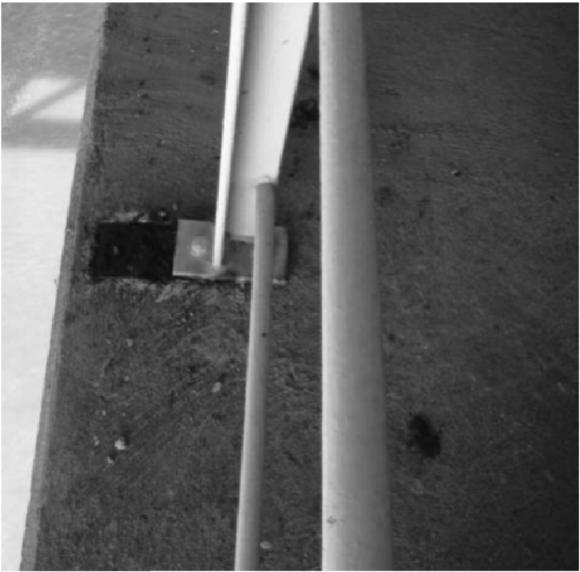
FAILED ANCHOR BOLTS AT SAFETY RAILING
