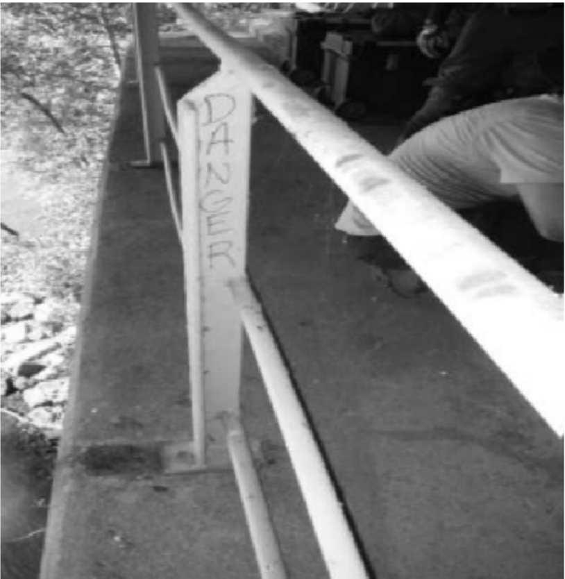
FAILED ANCHOR BOLTS AT SAFETY RAILING
